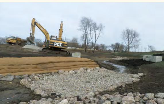
The geotextile fabric encapsulates the soil lift and provides structure and stability while the vegetation becomes established. Once established, the root systems of the willows and other vegetation stabilize the bank and decrease the speed of water flowing through the stream, reducing erosion of the streambank.
